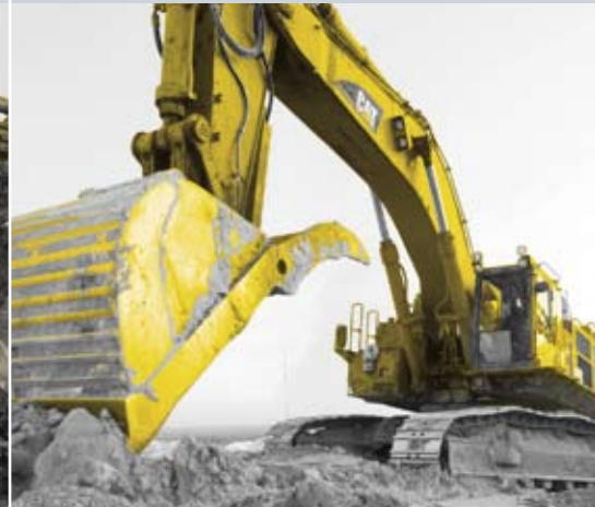
» Caterpillar Excavator, working tailings - Albian Sands
