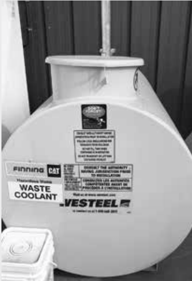
All tanks for liquid waste from maintenance are inspected regularly and are equipped with controls to prevent spills.
